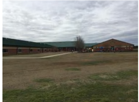
3). North Elevation - Jan 11, 2017
