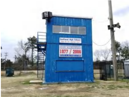
1). North Elevation - Jan 11, 2017
