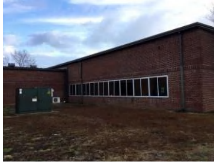
2). North Elevation - Jan 11, 2017
