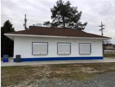
1). North Elevation - Jan 12, 2017
