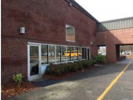
4). North Elevation - Jan 11, 2017
