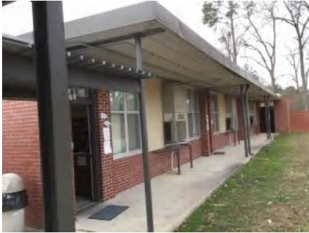
1). North Elevation - Jan 06, 2017
