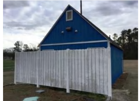
3). North Elevation - Jan 12, 2017
