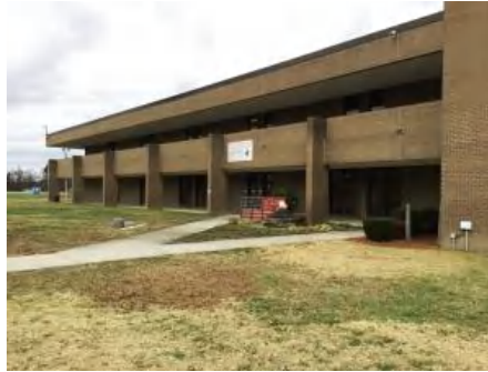
2). Southwest Elevation - Jan 11, 2017
