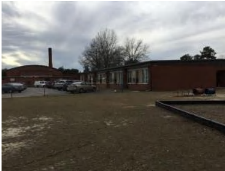
4). North Elevation - Jan 12, 2017
