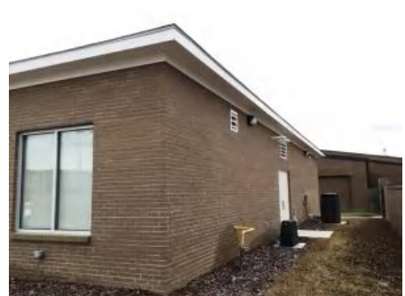
3). North Elevation - Jan 13, 2017
