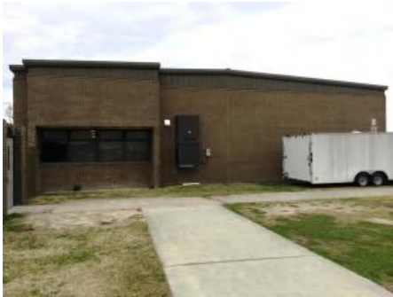
4). East Elevation - Feb 13, 2017
