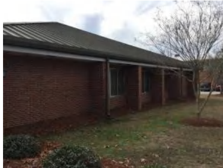
2). North Elevation - Jan 11, 2017
