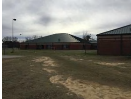
2). North Elevation - Jan 11, 2017
