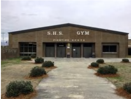
1). Southwest Elevation - Jan 11, 2017
