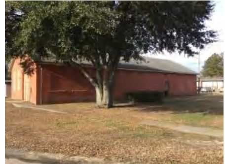
3). West Elevation - Feb 21, 2017
