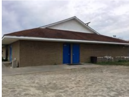
2). North Elevation - Jan 11, 2017
