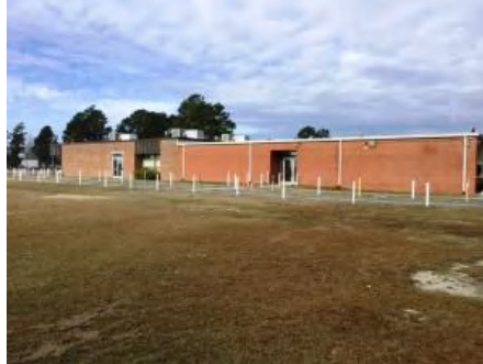
2). South Elevation - Feb 10, 2017
