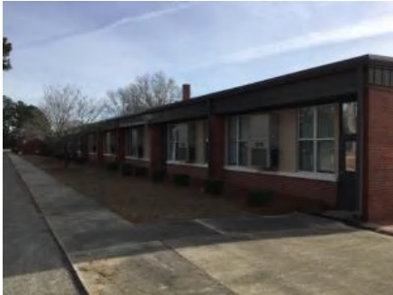
1). Northwest Elevation - Jan 10, 2017
