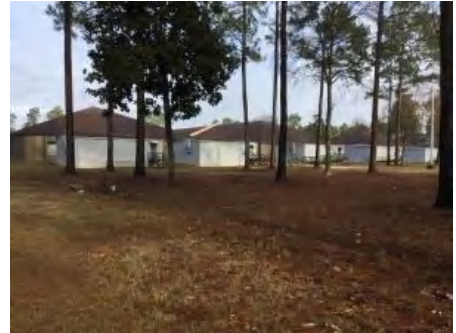
3). South Elevation - Feb 15, 2017
