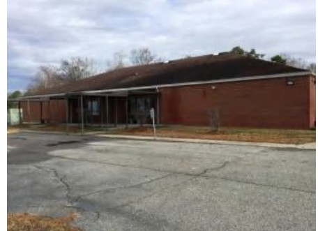
3). West Elevation - Feb 10, 2017
