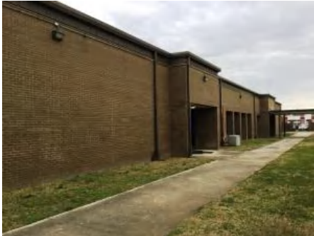
1). West Elevation - Feb 13, 2017
