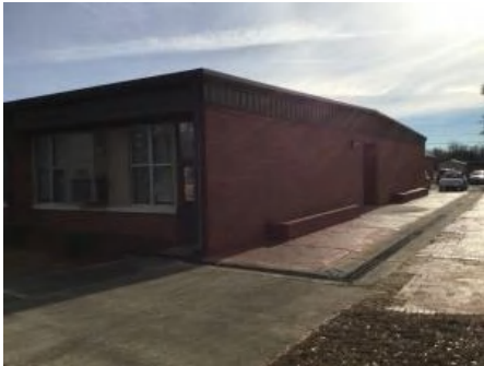
4). Southwest Elevation - Jan 10, 2017
