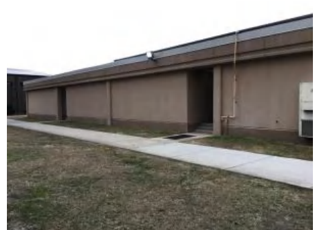
3). Southwest Elevation - Feb 14, 2017
