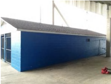
4). North Elevation - Jan 10, 2017
