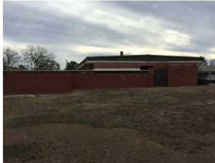
2). North Elevation - Jan 11, 2017
