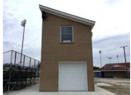
3). Southwest Elevation - Jan 12, 2017
