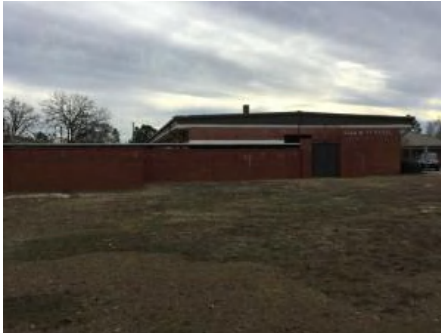
1). North Elevation - Jan 11, 2017
