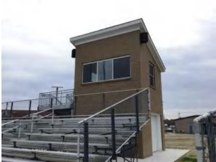
4). Northwest Elevation - Jan 12, 2017
