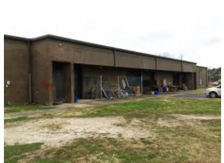
3). North Elevation - Feb 13, 2017
