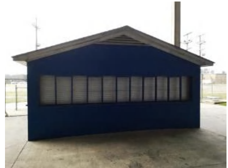
3). North Elevation - Jan 10, 2017
