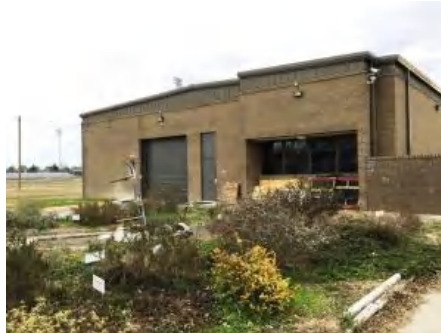
2). Northwest Elevation - Feb 13, 2017
