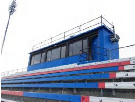
1). North Elevation - Jan 10, 2017
