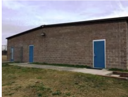
2). North Elevation - Jan 11, 2017
