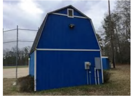
3). North Elevation - Jan 12, 2017
