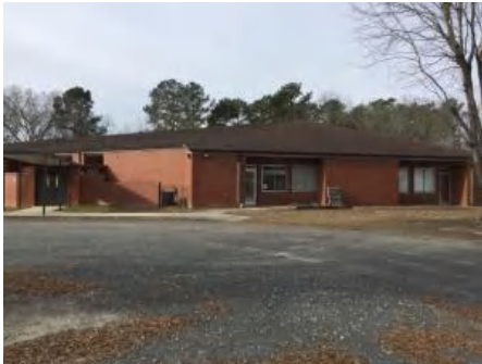
4). North Elevation - Jan 10, 2017
