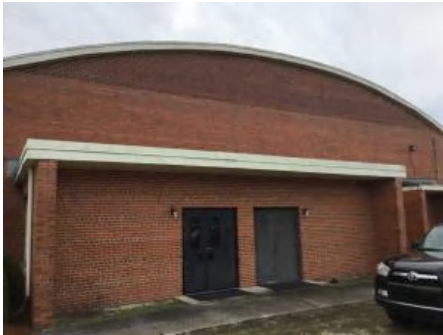
4). North Elevation - Jan 11, 2017
