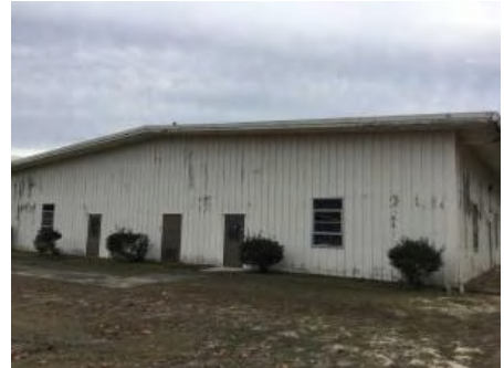
3). North Elevation - Jan 11, 2017
