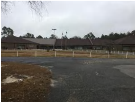
4). West Elevation - Feb 15, 2017
