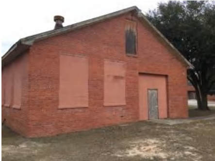
1). South Elevation - Feb 21, 2017
