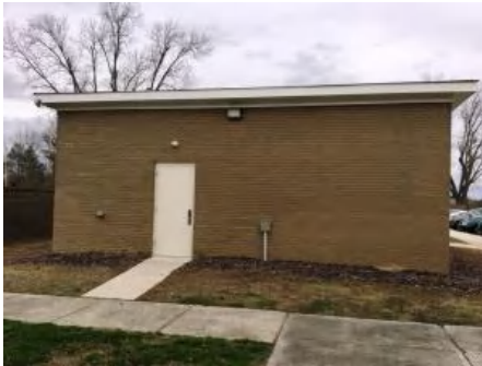
4). Southwest Elevation - Jan 13, 2017
