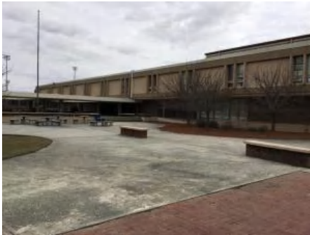
4). North Elevation - Jan 11, 2017
