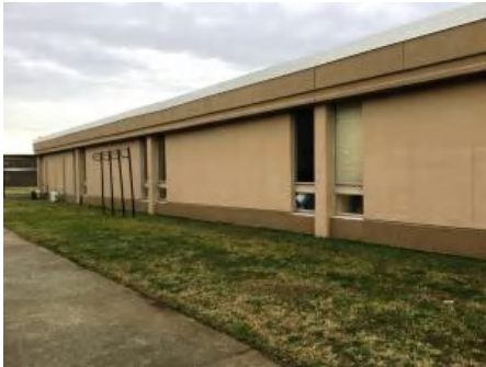
4). Northeast Elevation - Feb 14, 2017
