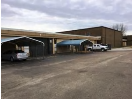
1). North Elevation - Feb 14, 2017
