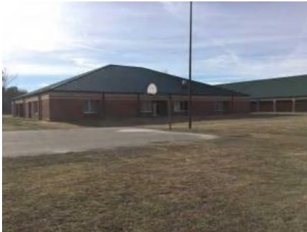
4). North Elevation - Jan 11, 2017
