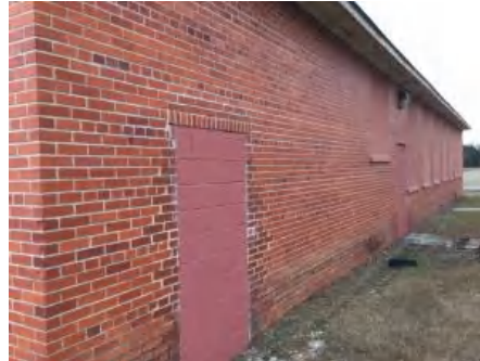
2). East Elevation - Feb 21, 2017
