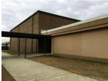
2). West Elevation - Feb 14, 2017
