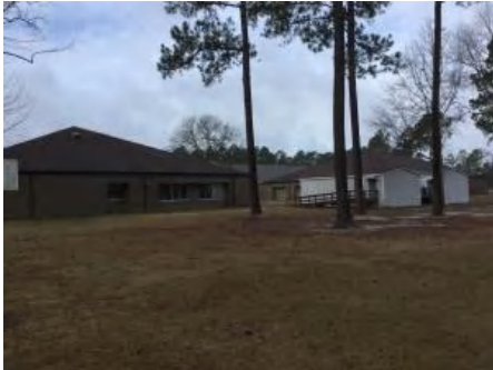
1). East Elevation - Feb 15, 2017
